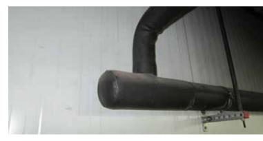
Figure 12. Pipe insulation in good conditions.
